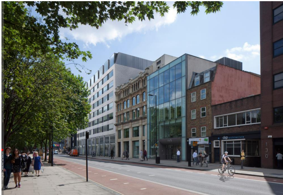
Image 12: Proposed development alongside the locally listed building fronting onto Old Street.
