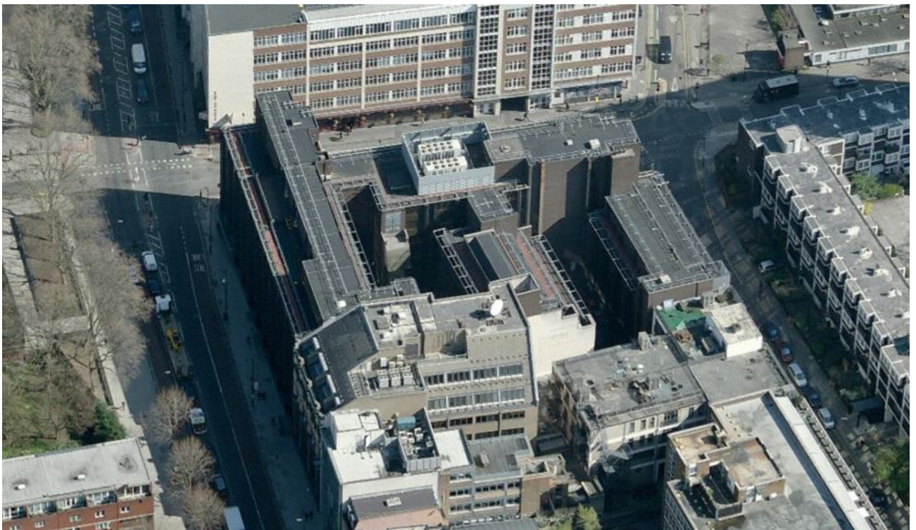
Photo 4: Aerial view from West
