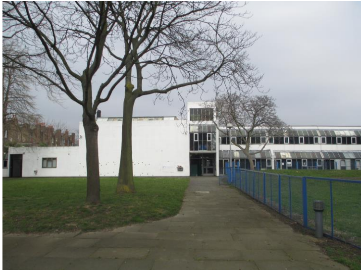
Photograph 5: The southern elevation of the school
