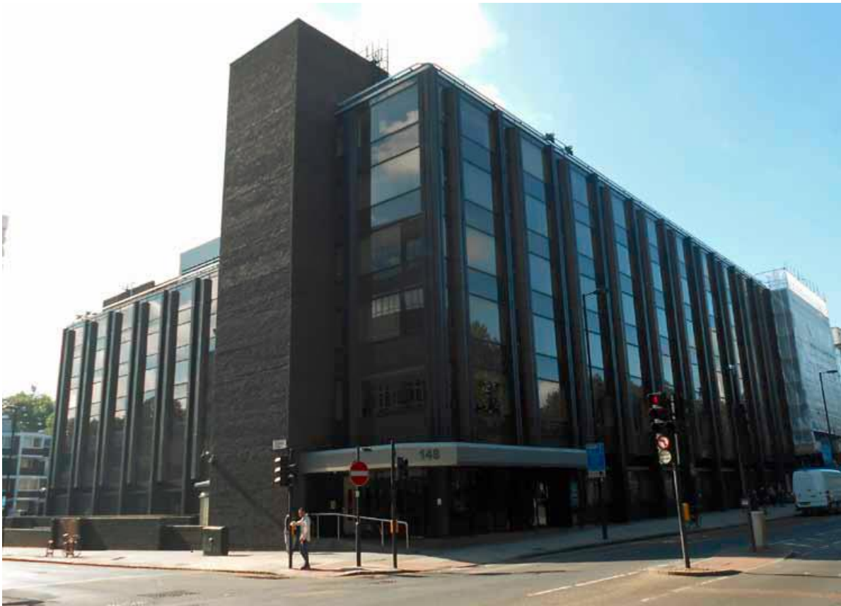
Photo 5: Front and Side Elevations fronting Old Street and Bunhill Row respectively
