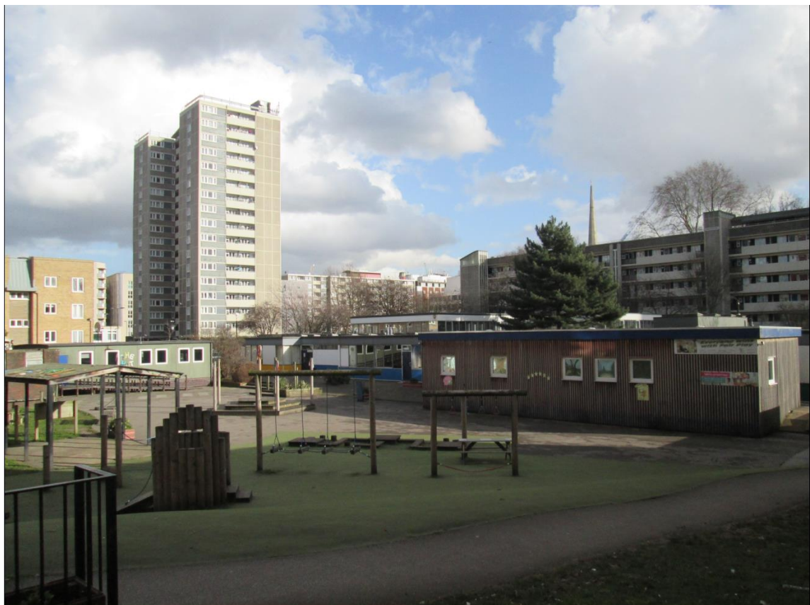
Image 4: View of north playground and north elevation of school building.
