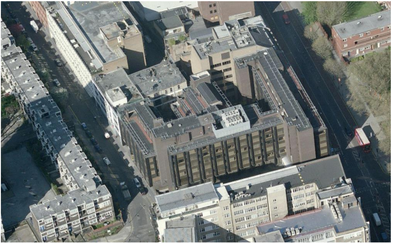
Photo 3: Aerial view from East (looking at the Bunhill Row frontage)
